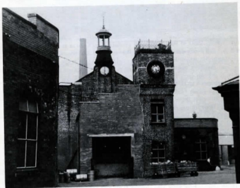
Bealey's Bleachworks, Radcliffe, showing wind indicator on tower (left) for favourable release conditions for poisonous gases, from their acid plant.
